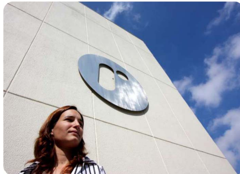
Centro de Serviços Afragade 1 Service Center Afragade 1
